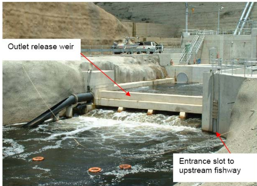
Figure 14 - Entrance to the trapping area and hopper (looking upstream from within the hopper approach channel) (DPIF 2008)
