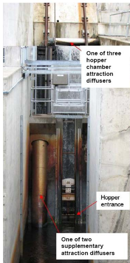
Figure 14 - Entrance to the trapping area and hopper (looking upstream from within the hopper approach channel) (DPIF 2008)
