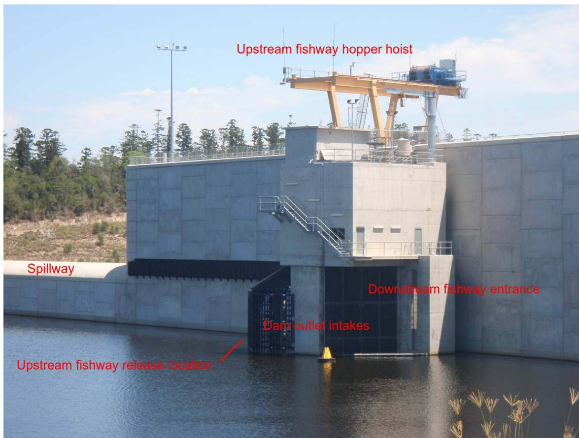
Figure 43 - Proximity of upstream fishway hopper release site to dam spillway, outlet intakes and downstream fishway entrance (J. Tait, December 2008)
