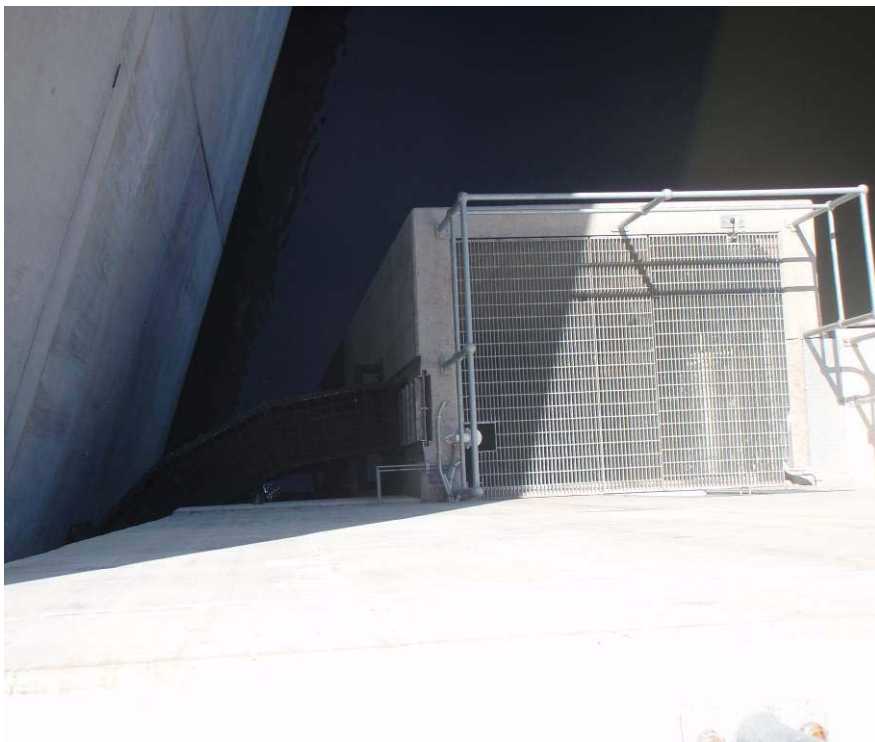
Figure 8 - Passage or “flume” joining to the inlet chamber of the downstream fishway (J Tait, December 2008)
