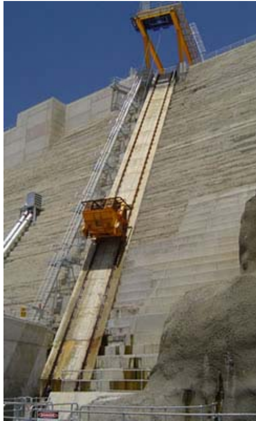
Figure 17 - Paradise Dam upstream fishway hopper traveling over the dam wall (SunWater, ca 2006)
