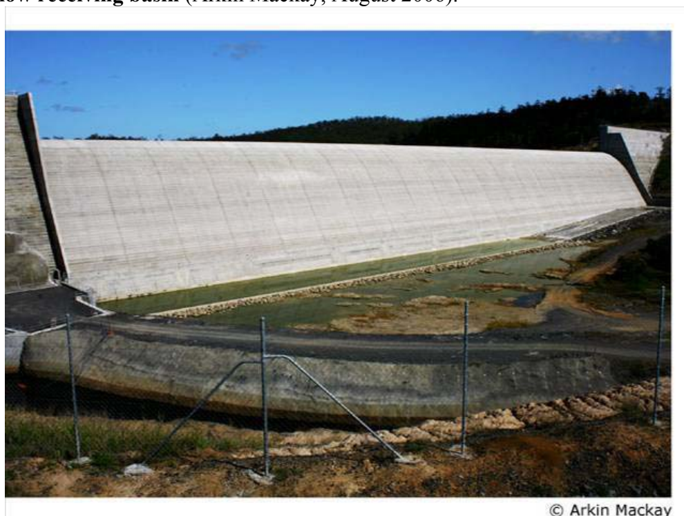
Figure 10 - Paradise Dam stepped spillway viewed from downstream showing shallow receiving basin (Arkin Mackay, August 2006).
