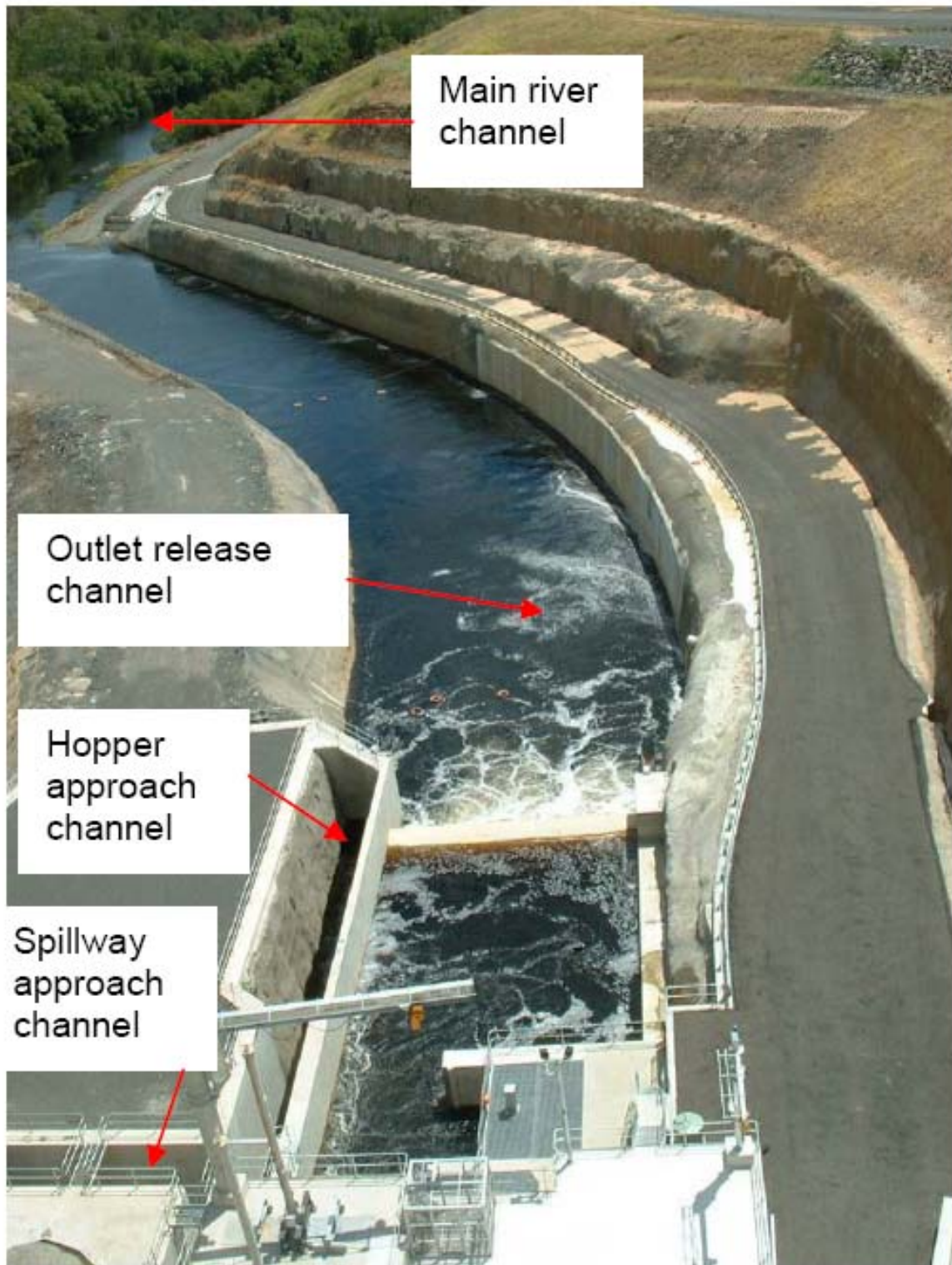
Figure 12 - Paradise Dam outlet release channel and upstream fishway approaches (DPIF 2008)
