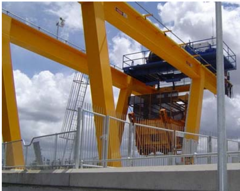
Figure 17 - Paradise Dam upstream fishway hopper traveling over the dam wall (SunWater, ca 2006)
