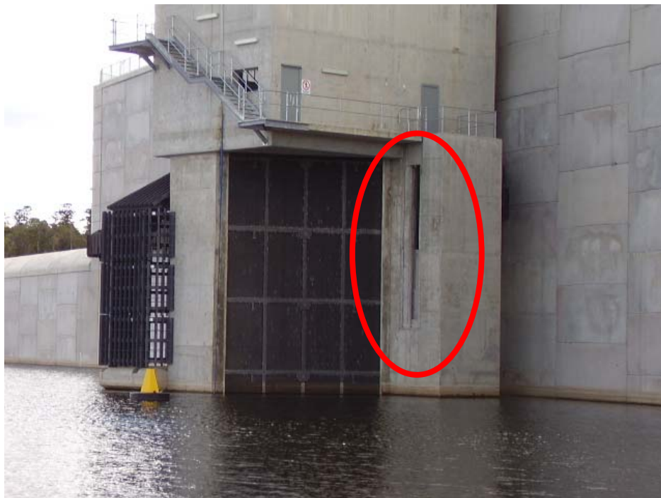
Figure 6 - Close-up of dam outlet works showing downstream fishway entrance (circled) above water (R Currie, 11 May 2008)
