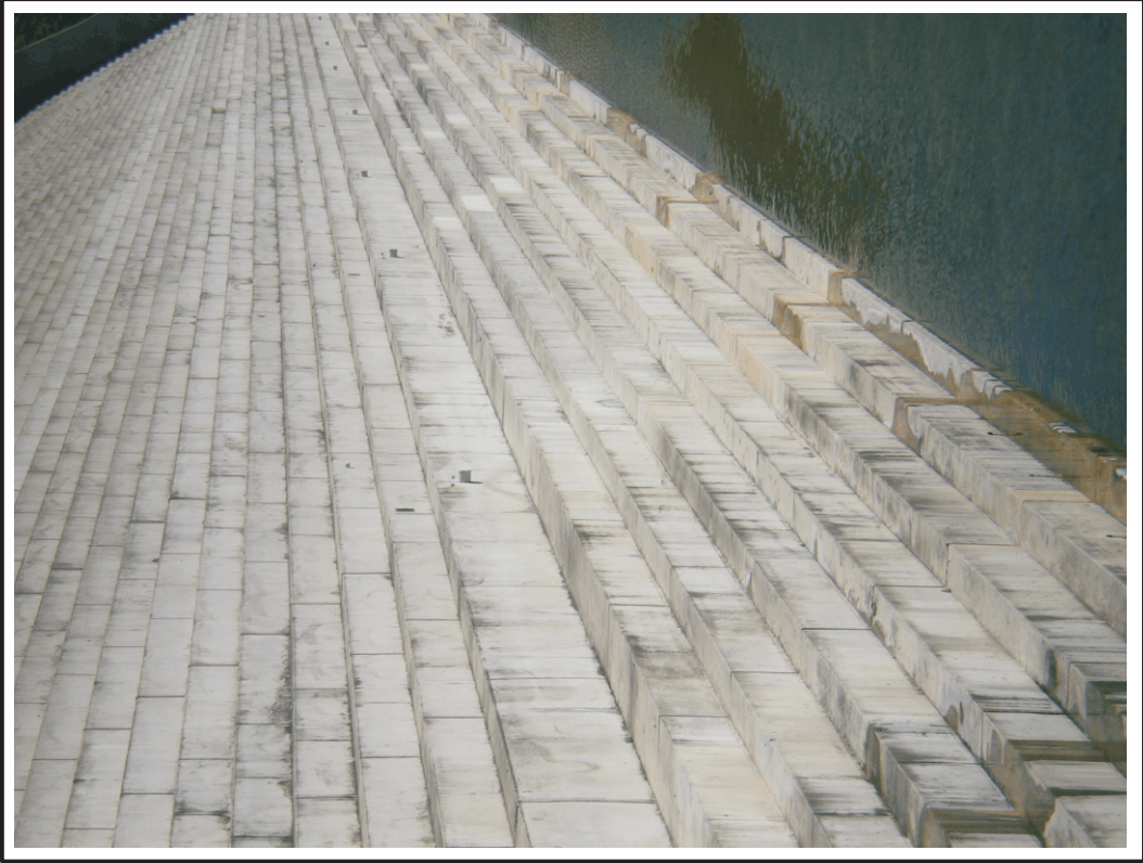
FIGURE 17(a) VIEW OF STEPPED SPILLWAY & PART OF STILLING BASIN
