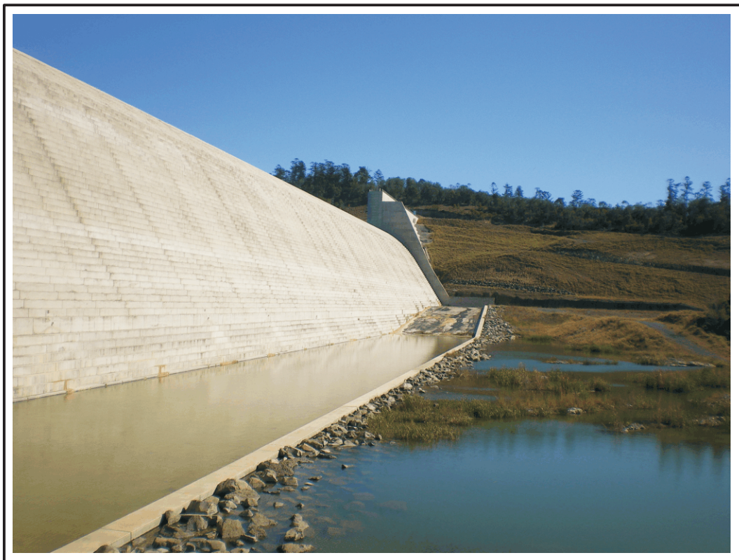
FIGURE 2(b) VIEW SPILLWAY & STILLING BASIN
