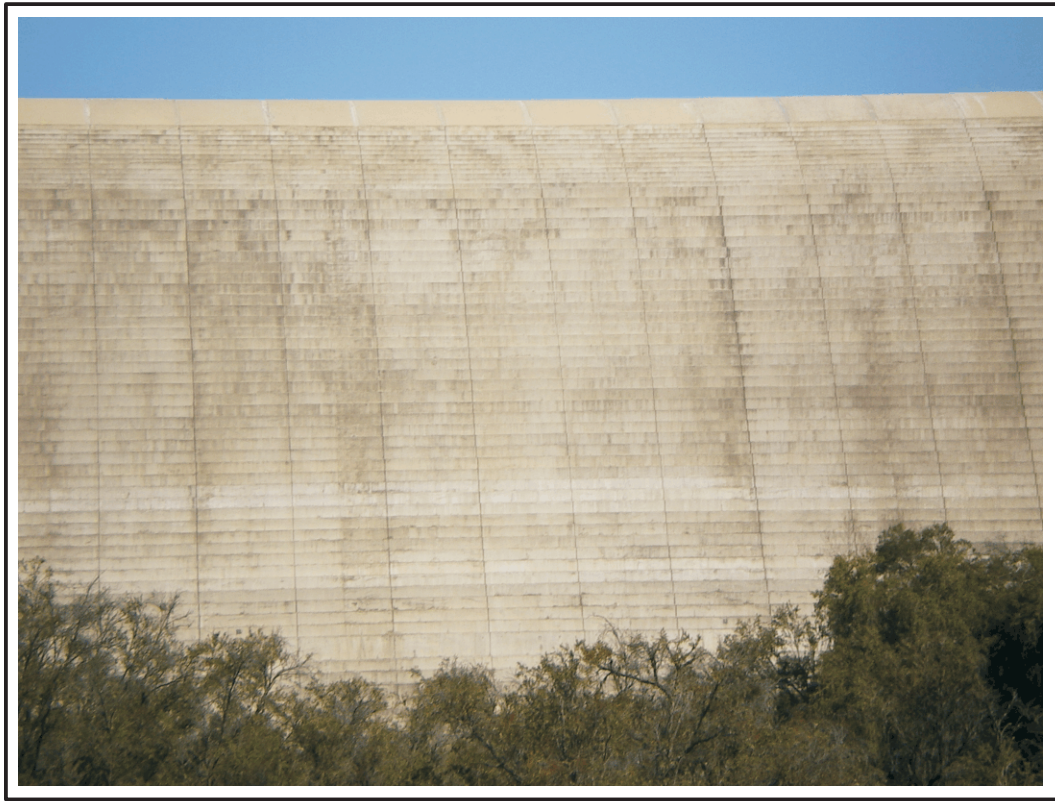
FIGURE 2(a) VIEW OF STEPPED FACE OF SPILLWAY
